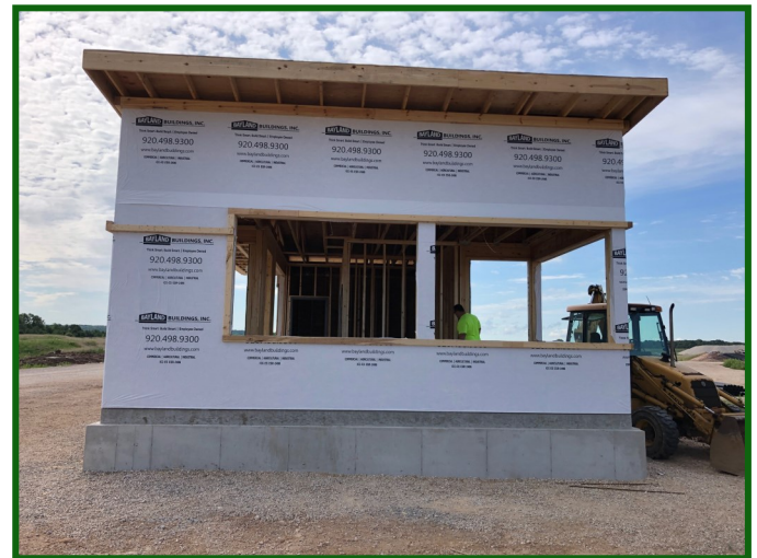
Scale House construction continues
