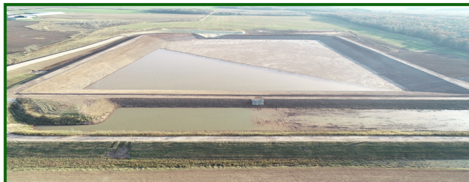
Main South Landfill excavated cell
