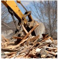
Contractors, waste haulers and shingle processors play a key role in providing sorted shingle scrap to asphalt plants with minimum contamination from other materials. Contaminants in roofing debris can include: asbestos from flashing; fabrics; rolled roofing; mastic; pre-1973 shingles; wood; metal; cardboard; plastic packaging; and, shingle nails, which all affect pavement acceptability.
