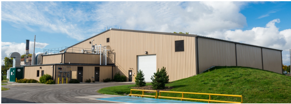
UW-Oshkosh's Biodigester Building
